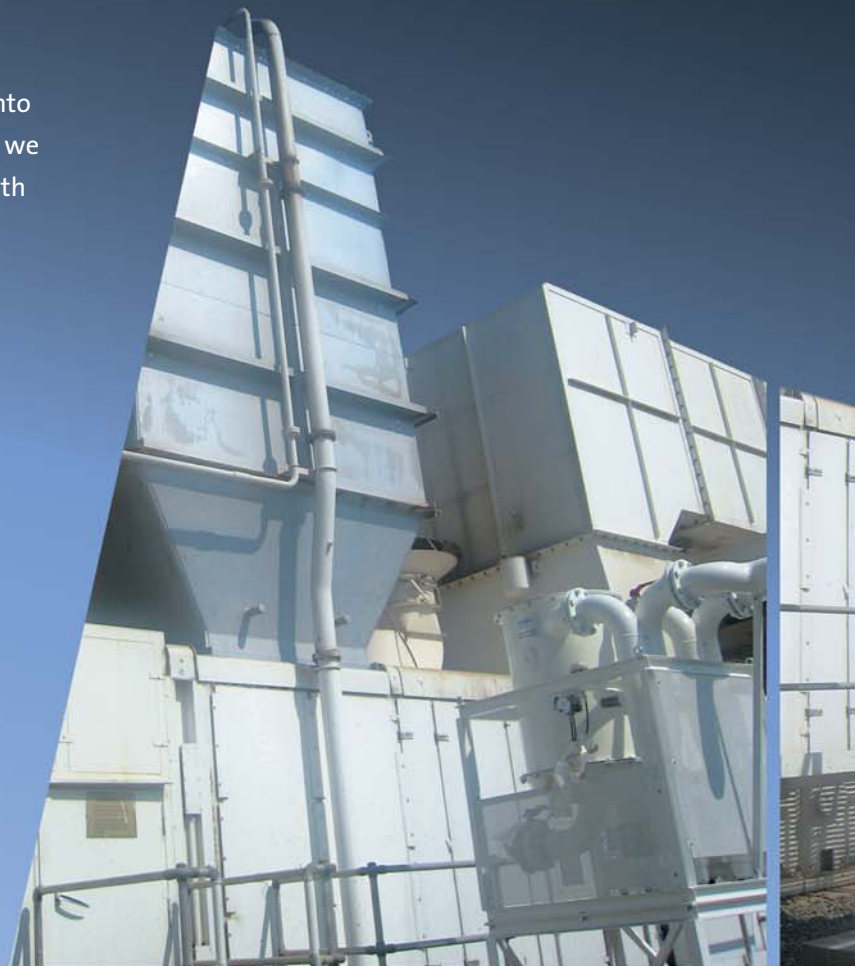
Successful project: Oil mist separator from FRANKE FILTER at gas turbines in Abu Dhabi
